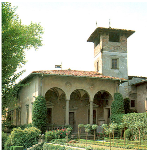
Villa Zavaritt (foto Wikipedia)
